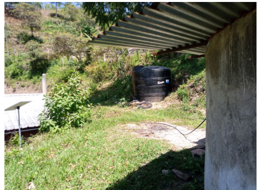
Black 1,500 gallon water tank, and the wall of the cement tank in the foreground
