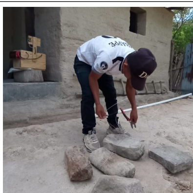
Homeowner preparing rocks to mount solar panel on roof
