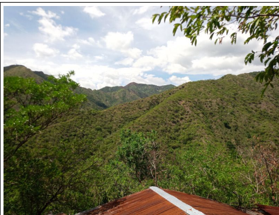
Roof view of a home where we will place a solar panel
