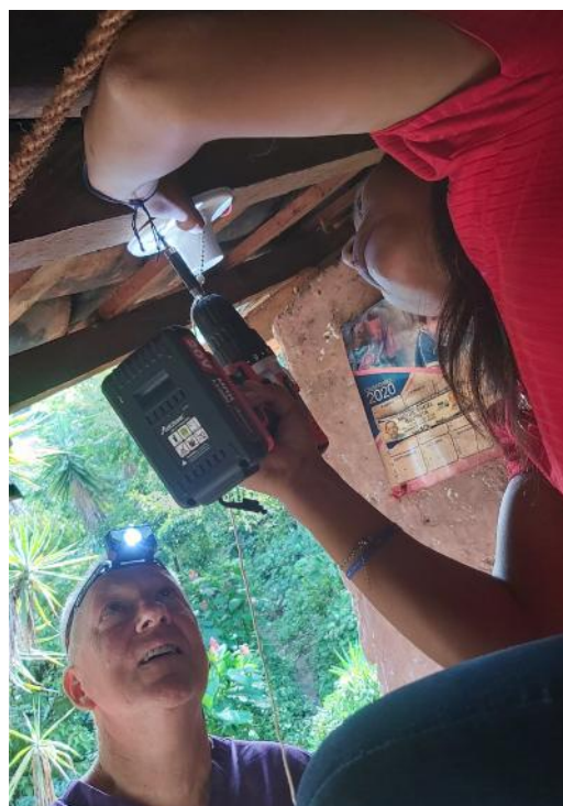
Ana installing light socket as Doug guides
