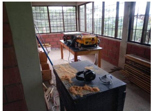
The Volunteer house porch turned into a workshop
