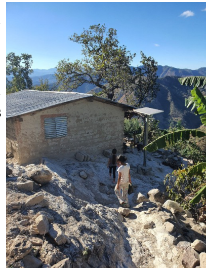
Solar system installed 5 years ago by another group at an isolated home
