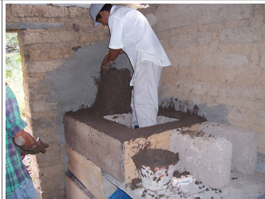
Placing mud around chimney tiles
