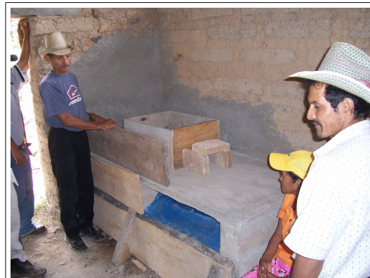
Inner form in place and positioning outer form
