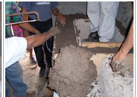
Placing barb wire in form
