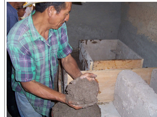
Placing mud in form
