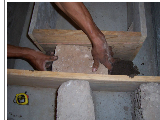
Placing top brick in place
