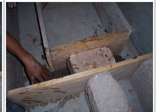
Placing mud around bricks to seal in place
