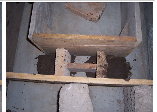
Wood spacer holding bricks in place
