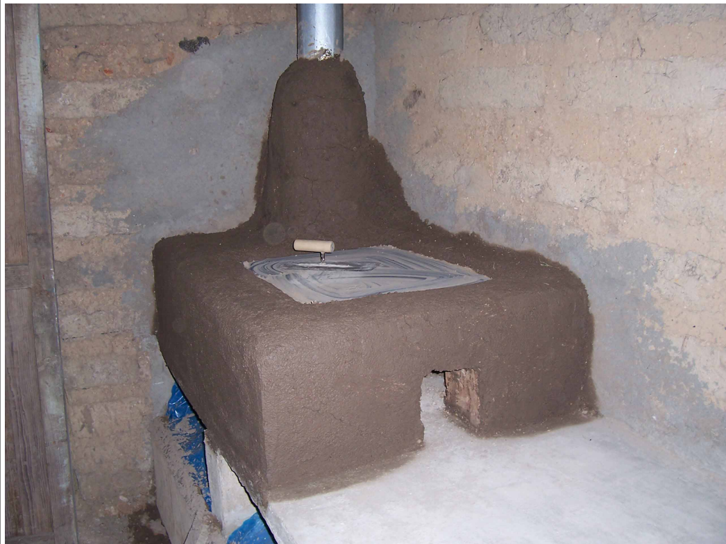
Finished stove drying after removal of forms and placement of Plancha
