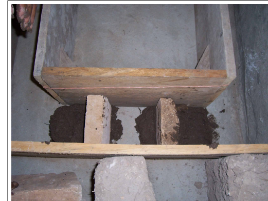
Placing bricks in place for air-wood entry
